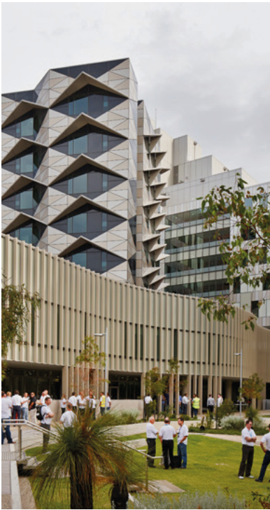
Fiona Stanley Hospital, Perth, Australia (2014)
