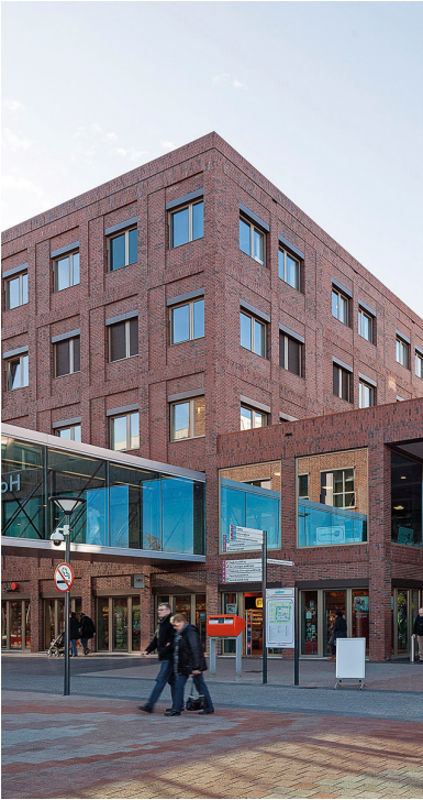
Maasstad Hospital, Rotterdam, The Netherlands (2011)
