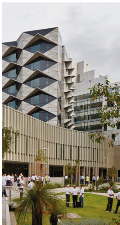
Fiona Stanley Hospital, Perth, Australia (2014)
